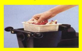
Cleaning the skimmer & Pump Baskets regularly is important to the overall maintenance of your swimming pool. Clogged baskets mean your pump has to work harder to try to cycle the water. This can decrease the life and stress the seals in your pump.
